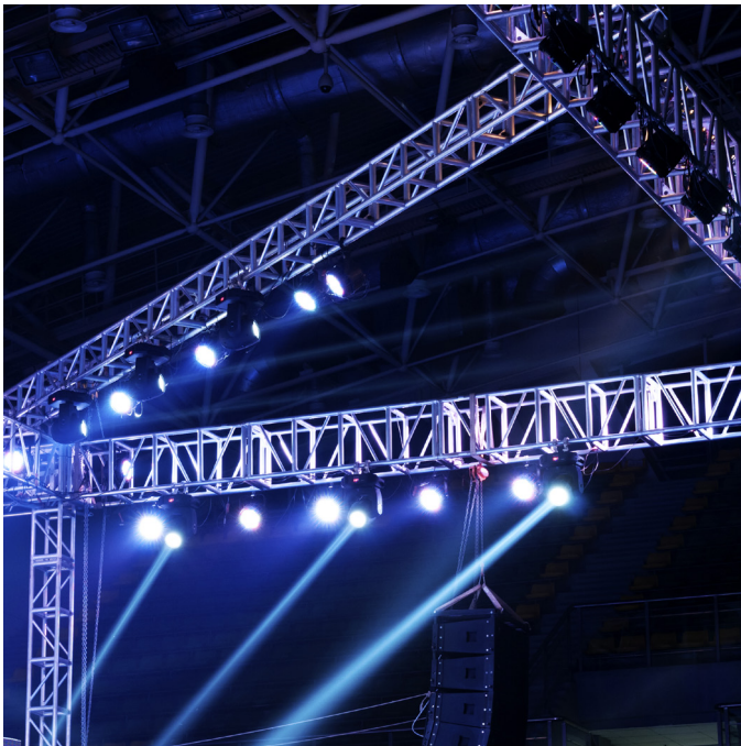
Figure 01 – Stadium and Stage LED lighting quickly deploying.
