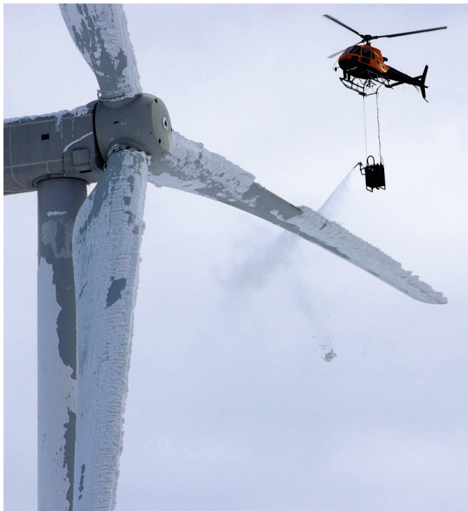
Picture 04: Airborne de-icing by helicopter projecting hot-water on the frosted blades (Picture: PRBX / Courtesy of Energiforsk)
