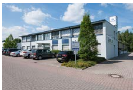
EPLAX headquarters in Bremen
